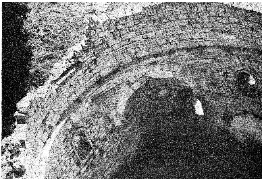
Fig. 5. Example of a "Bosnian dome" built of small blocks of roughly cut stone without the use of pots. Beğluk Cami, Livno, Bosnia.
